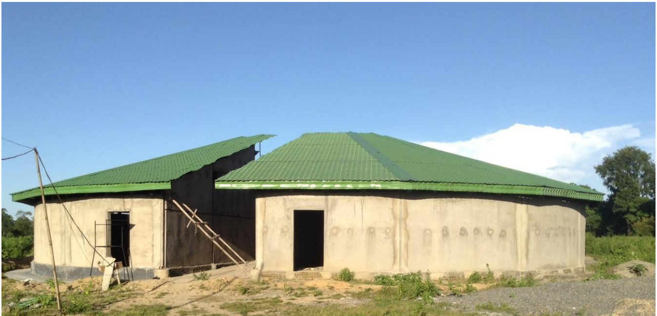
Figure 15: Partly constructed main hub of the KDP
